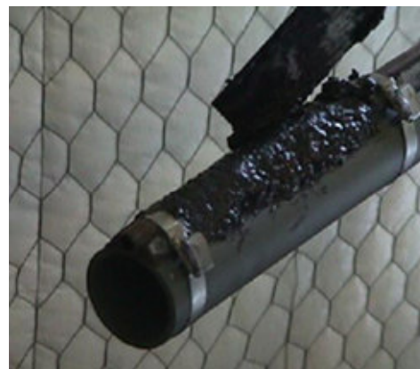
Typical hand trowel application
